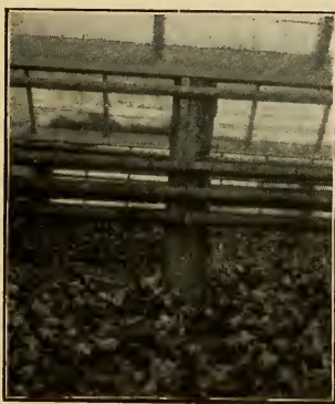
18.—Fastening pipes to posts by bent-wire nails
